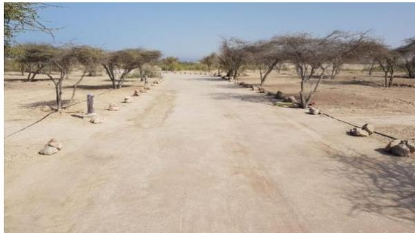
**Project Description:** The areas were constructed by creating a stabilized layer which was compacted then shaped properly to ensure for drainage. The surface was then made smooth and ready for the application of the EBS Surface Seal, which seals and protects the surface from erosion, cracking and any form of deterioration. All work was completed by Soil Solutions and Scan Construction.
